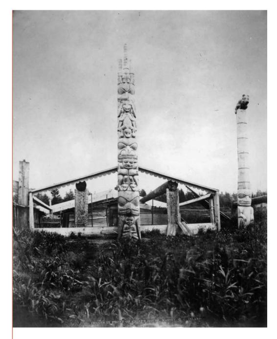
**Figure 2:** Star House was built in Old Massett between about 1878 and 1881. Oregon Hastings' 1878 photo of Massett shows Anetlas' house with only the interior house posts in place, and the frontal pole already raised. (Courtesy Royal British Columbia Museum, PN5540)
